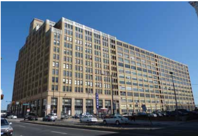
Older industrial buildings are physically suitable for loft conversion in the Redevelopment Loft Zone.
